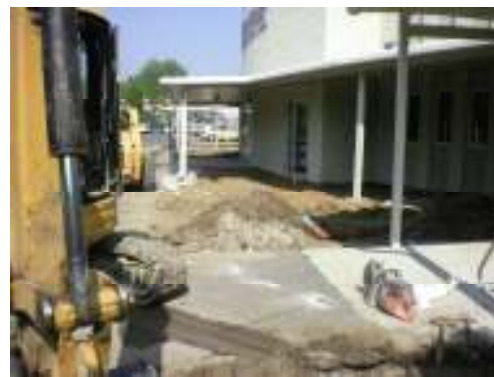
Extensive work to prevent further damage to the corps building began on September 30.
